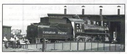
was balanced correctly, it could be turned by two to six men. Larger turn-tables were driven by either steam or electric motors. The turn-table allowed the engine to be moved into a particular stall in the roundhouse - the number of stalls depending on the needs of the railroad at that location.
