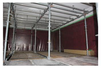
This picture captures work underway in the dining room. Carefully constructed supports were used to secure ceilings of Bellevue House while plaster conservation specialists worked on them from the floor above.
