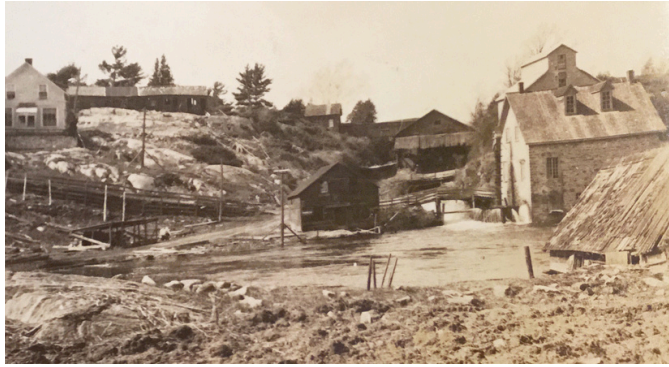
Bedford Mills c 1920. The store is upper left, sawmill in middle, hydro plant in former gristmill building on right.
